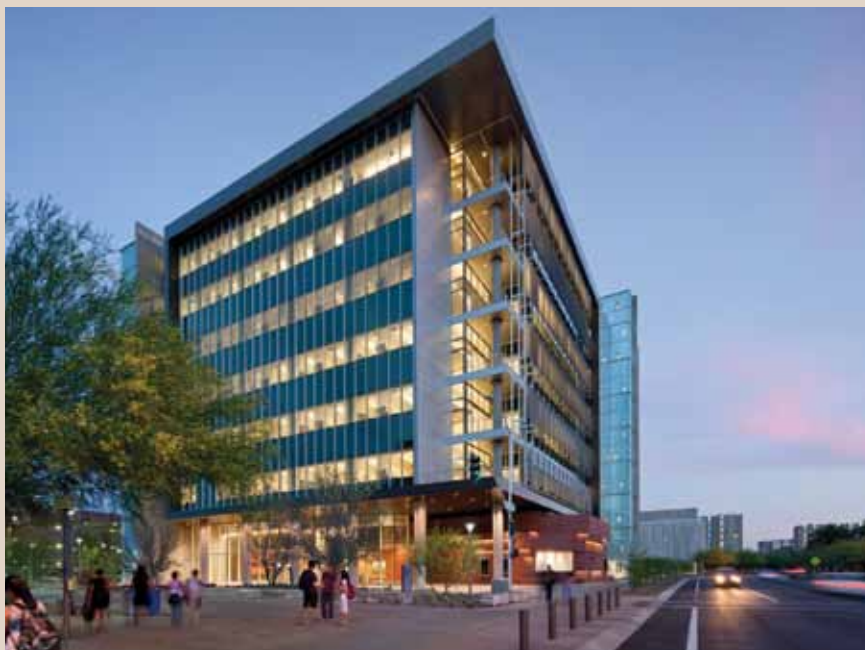
Arizona State University's newly opened LEED Gold certified Interdisciplinary Science and Technology IV (ISTB 4) research building is the single largest research building at ASU, with 298,000 square feet of premier high-technology research laboratories and office space.
