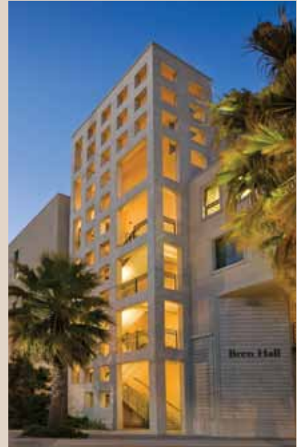
Bren Hall at UC Santa Barbara, is the nation's first building to earn two LEED Platinum certifications—one for LEED NC in 2002 and one for LEED: EBOM in 2009.
