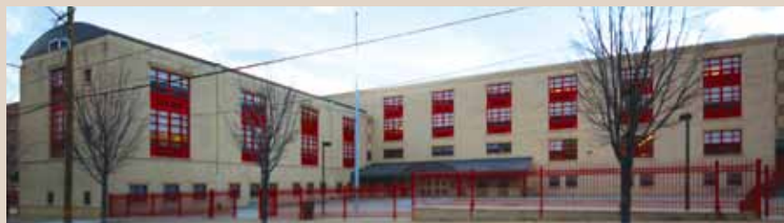
Built in 1997, the 114,000 square-foot, LEED:EBOM certified, Thurgood Marshall Elementary School, serves more than 700 students, grades pre-K through 8, with over 100 teachers and staff members.
