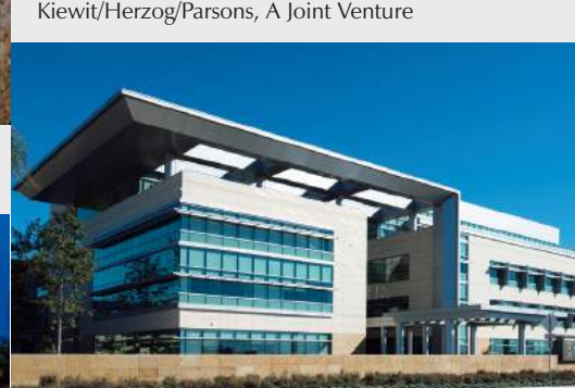
Partnering (2014) | Naval Hospital Camp Pendleton | Camp Pendleton, CA | Clark/McCarthy, A Joint Venture
