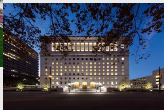
Building Renovation $11M to $199M (2015) | Hall of Justice - Repair & Reuse Project | Los Angeles, CA | Clark Construction Group – California, LP
