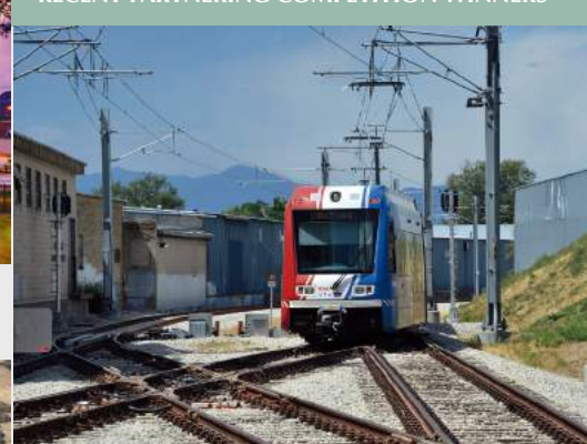
Partnering (2015) | Draper Light Rail Transit Design-Build Project | Sandy City and Draper, UT | Kiewit/Herzog/Parsons, A Joint Venture
