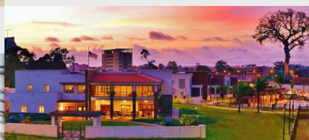
International (2015) | New U.S. Embassy | Malabo, Equatorial Guinea | Caddell Construction Co.
