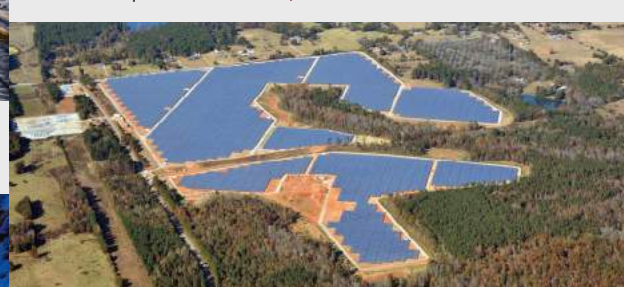
Utility Infrastructure New (2015) | Simon Solar Farm Photovoltaic Facility | Social Circle, GA | Crowder Construction Co.
