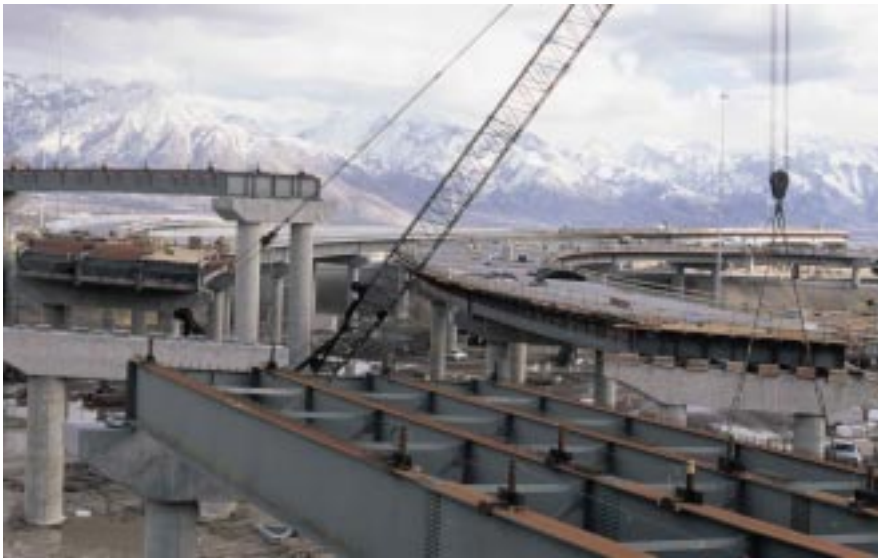
Bridge deck construction of the I-15/I-80 Interchange.
