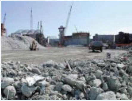
Concrete and rebar ready to be processed.
