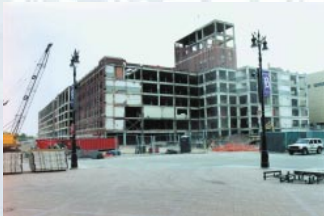
As part of the Ford Field stadium project, more than 25,000 cubic yards of concrete and more than 1,000 tons of structural steel were removed and recycled.
