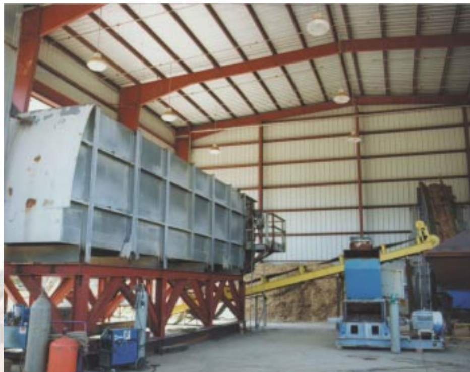
An up-close look at the “walking floor machine” that controls constant feeding of wood chips to the gasifier. The wood gasification process provides fuel to a steam boiler that drives a turbine, which in turn generates electric power for the facility.
