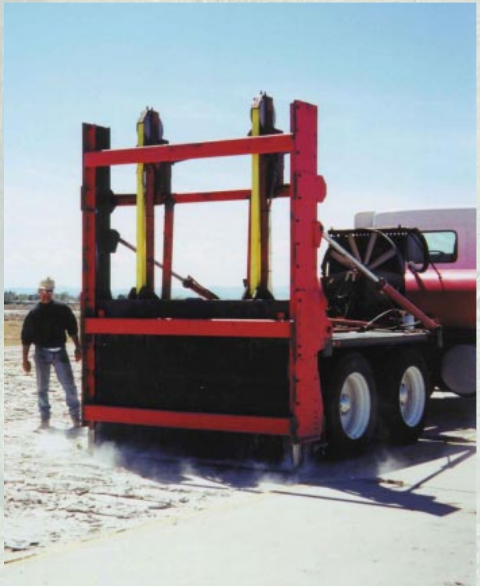
The 16,000-pound weight dropped by RMC's guillotine breaker makes the initial cracks in concrete runways averaging 24 inches thick.
