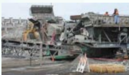
The on-site rock crushing operation used in Turner's immense recycling project.
