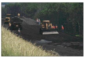
Above, for a \$51 million OTC project, AGC members Trumbull Corp. and National Engineering & Contracting Co. demolished and rebuilt the east- and west-bound bridges over the Cuyahoga River. Kurtz Bros. supplied around 54,000 tons of spent foundry sand for a terraced, land-scaped embankment measuring 450 feet in length by 55 feet in width and depth.
