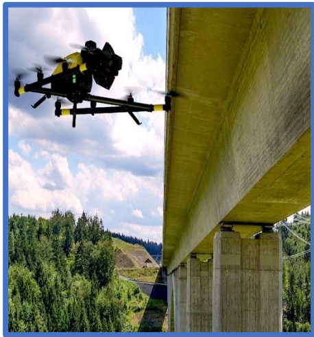
Figure 2 - Drone inspects bridge condition
