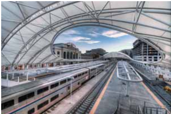
Denver Union Station Transit Improvements Kiewit Infrastructure Co
