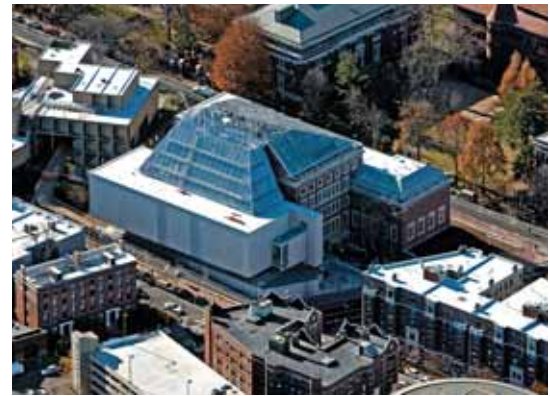
32 Quincy Street Expansion and Renovation Skanska USA Building
