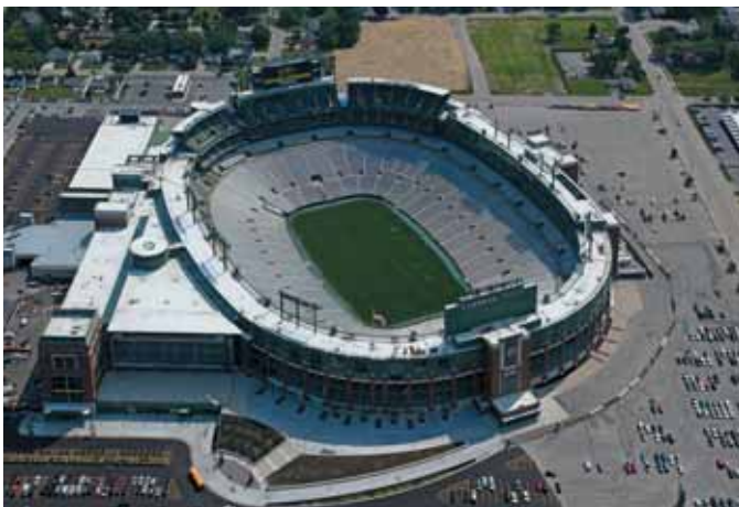
Lambeau Field North & South End Zone Stadium Improvements Miron Construction Co
