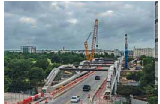
West 7th Street Bridge Sundt Construction, Inc.
