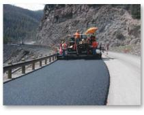
production is at temperatures ranging from 30 to 120 degrees lower than hot mix. In most cases, the lower temperatures result in significant cost savings and reduced greenhouse gas emissions because less fuel is required. WMA also has the potential to extend the construction season, allowing projects to be delivered faster. By 2009, more than 40 States constructed WMA projects, with 14 adopting specifications to accommodate WMA.
