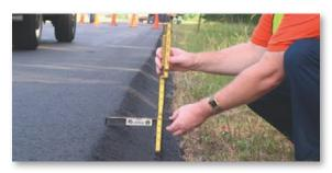
The asphalt Safety Edge provides a strong, durable transition even for vehicles that are particularly vulnerable, such as smaller, lighter cars. Even at higher speeds, vehicles can return to the paved road smoothly and easily. FHWA's goal is to accelerate the use of the Safety Edge technology, working with States to develop specifications and adopt this pavement edge treatment as a standard practice on all new and resurfacing pavement projects.
