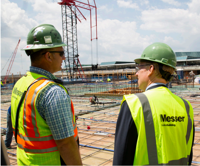
Messer Construction Company carpenter Mark Miracle showcases his company's $114 million design-build project to build a new terminal parking garage and an airport administrative building at the Nashville Airport to Tennessee Congressman John Rose (right).
