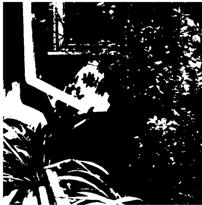
Downspout Disconnection
