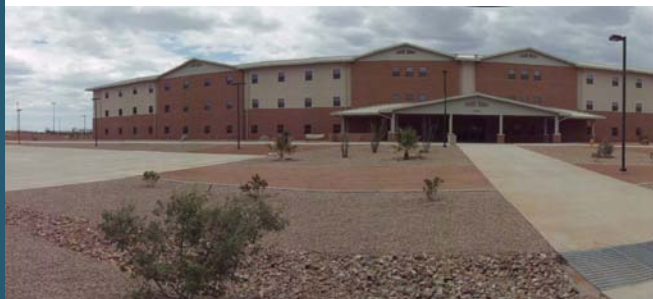
Fort Huachuca Advanced Individual Training Barracks Complex | Fort Huachuca, AZ | Sundt Construction, Inc.
