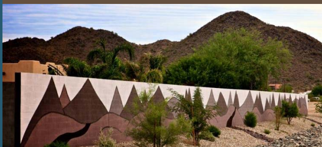
Happy Valley Road – 67th Avenue to Lake Pleasant Parkway | Peoria, AZ | Ames Construction, Inc., City of Peoria
