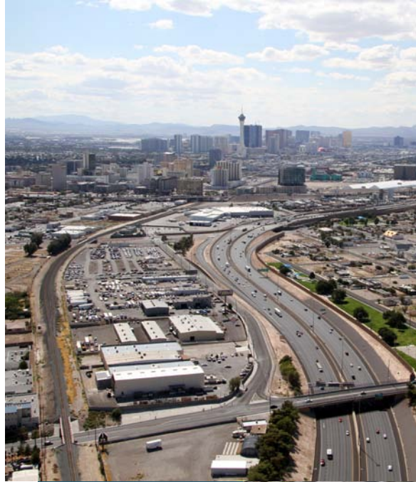
I-15 North Corridor Design-Build Project | Las Vegas, NV | a CH2M Hill/Las Vegas Paving Corporation Joint Venture
