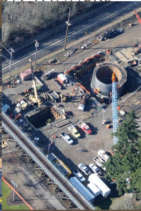
Lower Tualatin Pump Station | Tualatin, OR | Natt McDougall Company
