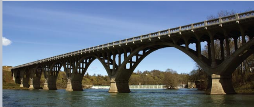
Build America Award: Highway Renovation | Oregon Highway 99 – North Umpqua River (Old Winchester) Bridge Rehabilitation | Douglas County, Oregon | Hamilton Construction Company
