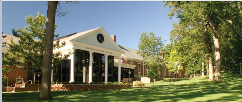
Build America Award: Construction Management Renovation | Kalamazoo College Hicks Center | Kalamazoo, Michigan | Miller-Davis Company
